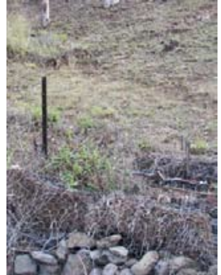
Use of hay bales and rocks makes a sediment trap for runoff from a spotted gum ridge.
