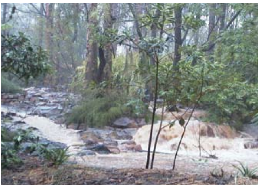
No erosion: The western drain on Dave and Pam Grubb's Laidley property during heavy rains in February 2001.
