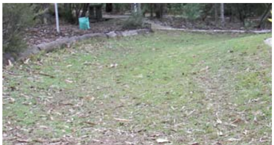
Spoon drain: A well grassed spoon drain on the Laidley property of Pam and Dave Grubb safely transfers water across the property.
