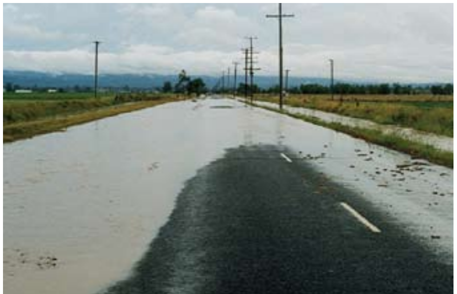
Keeping roads with a low profile is important to avoid concentrating flows.
