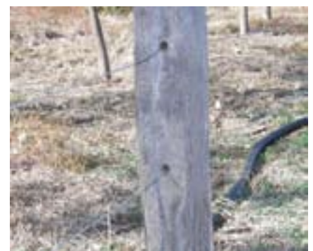
No catch – having 2 plain wires at the bottom of the fence reduces debris buildup.
