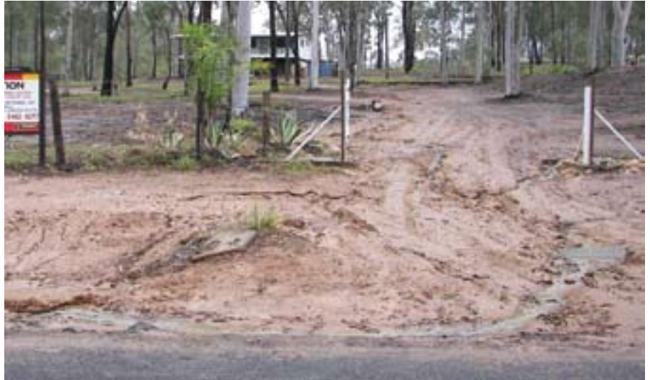
This farm track south of Gatton shows serious erosion and is contributing to sediment in waterways. The highly erodible soil creates difficulties. Better design could avoid most of the problems.
